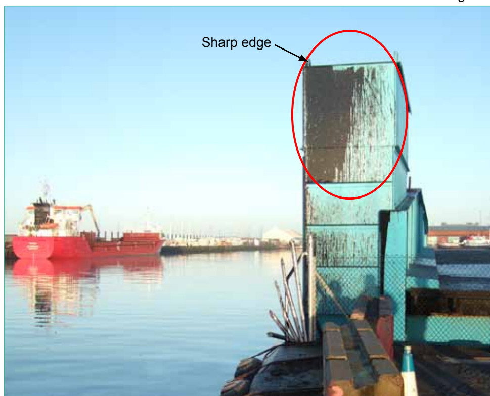
Swing bridge showing counterweight
